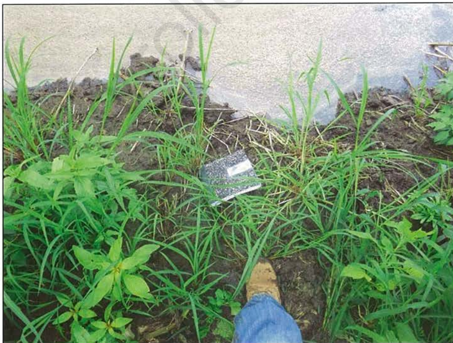
Photograph 34. Standing on the lower lagoon overflow spillway, I estimated the freeboard of the lagoon at approximately twelve inches (note the notebook for reference). Photo by A. D'Angelo; 12/14/16.
