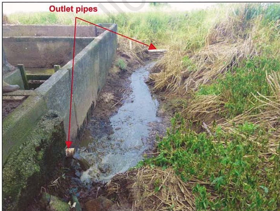
Photograph 24. View of the two pipes that drain separated liquid from the manure solids separation cells. Liquid from the cells surface flows, via an earthen conveyance channel, into the northwest side of the upper lagoon. Photo by A. D'Angelo; 12/14/16.
