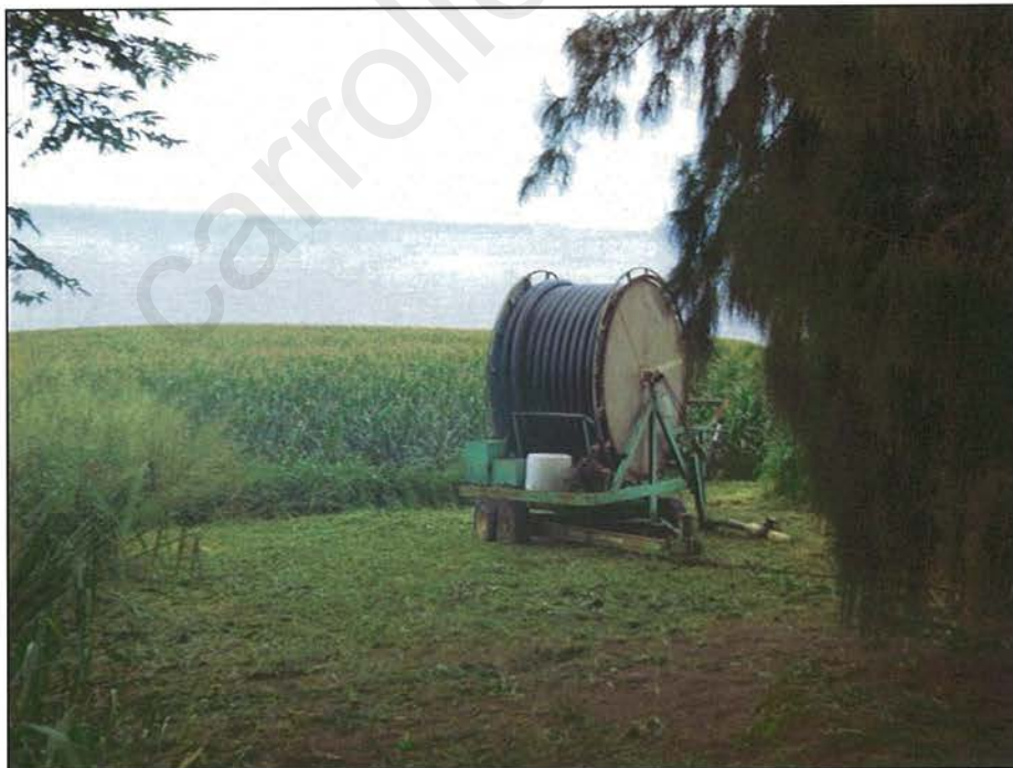
Photograph 30. View of one of the Facility's retractable irrigation distribution equipment which receives flow from the lower lagoon draw pumping system. Photo by A. D'Angelo; 12/14/16.
