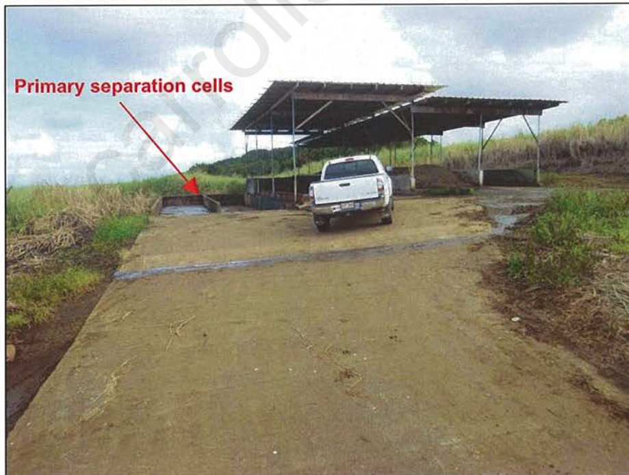
Photograph 22. View, facing east, of the Facility's manure solids separation cells located adjacent to the upper lagoon (refer to Figure 2). The uncovered cells on the left serve as the primary cells and liquid waste discharge points. Photo by A. D'Angelo; 12/14/16.
