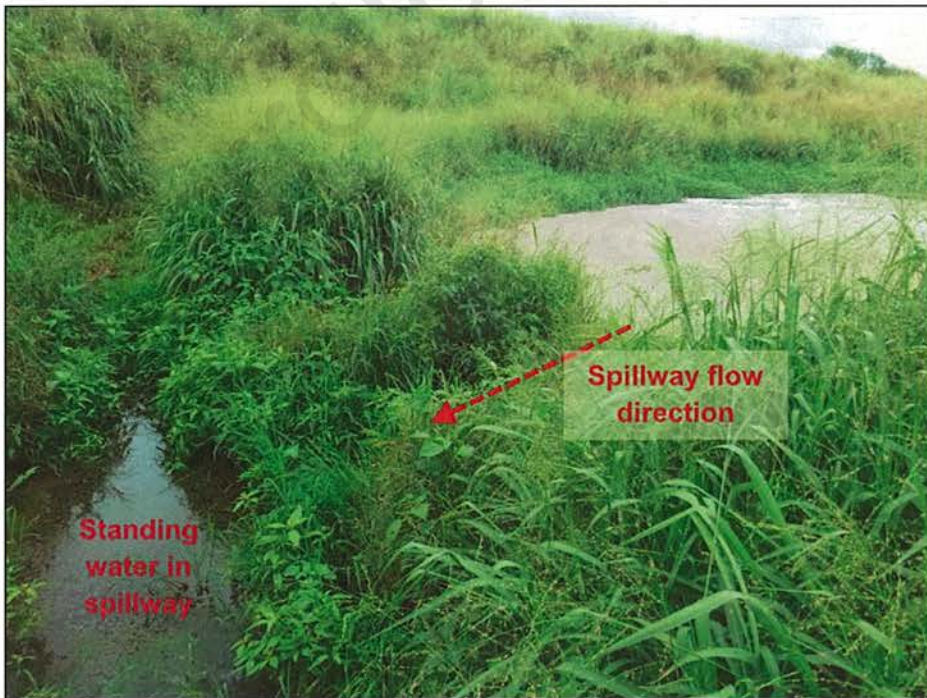
Photograph 32. View, facing southwest, of the lower lagoon overflow spillway. Note the presence of algae growth and standing water in the overflow spillway. Photo by A. D'Angelo; 12/14/16.
