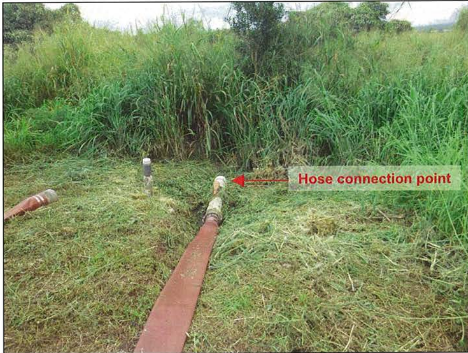
Photograph 29. View of the draw pumping system hose connection point to the Facility's irrigation system. Photo by A. D'Angelo; 12/14/16.
