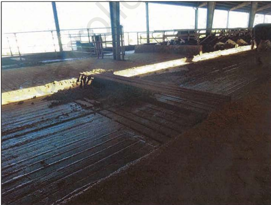
Photograph 8. View of the manure collection trough in the center of the lower freestall barn. The contents of the collection trough gravity flow into a collection pit located at the manure composting building, shown in Photographs 15 and 16. Photo by A. D'Angelo; 12/14/16.
