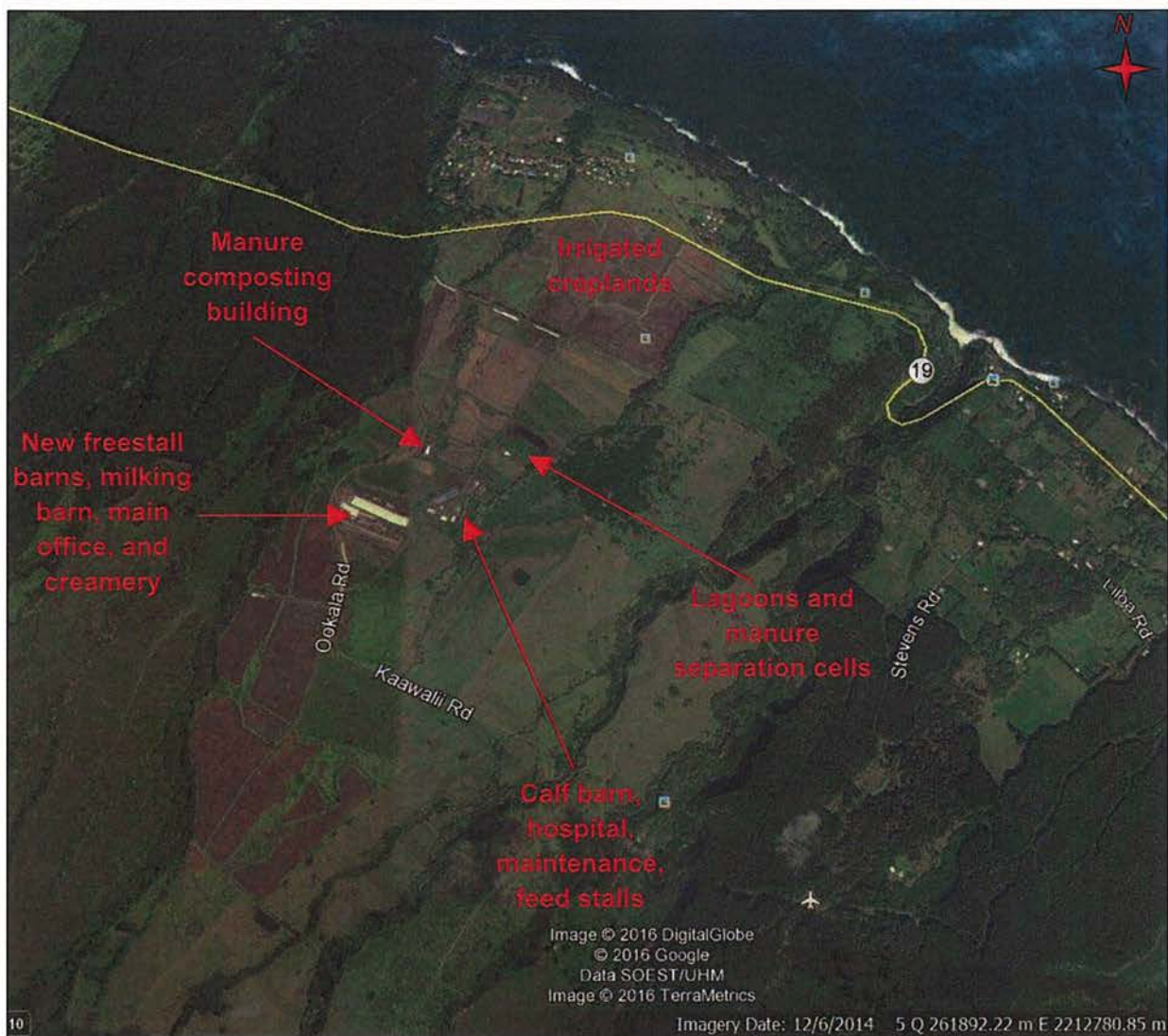
Figure 1. GoogleEarth aerial image of the BID Facility, imagery date December 6, 2014. The red arrows and callouts identify the various areas of the Facility visited during the inspection.
