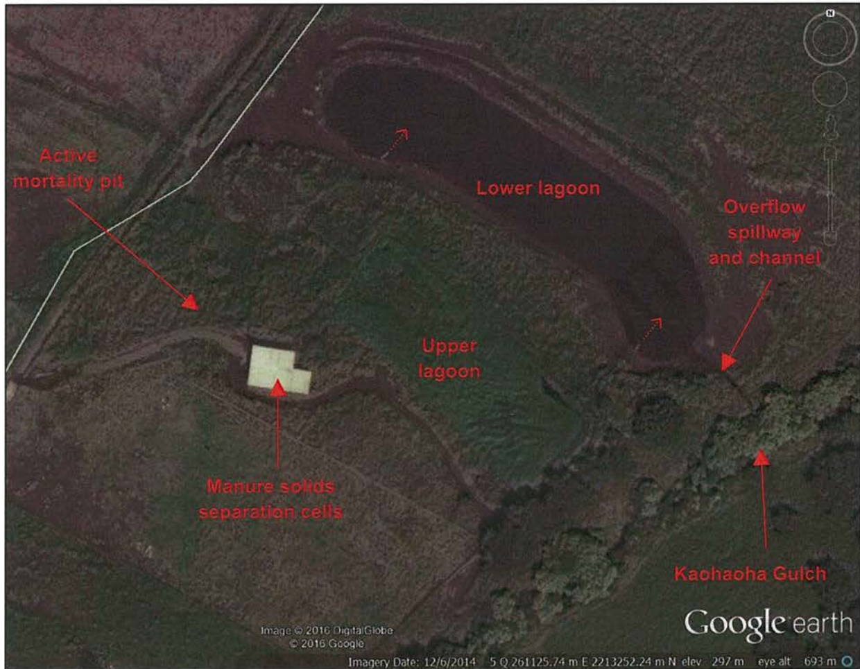
Figure 2. GoogleEarth aerial image of the BID manure separation cells and wastewater lagoons, imagery date December 6, 2014. The red arrows and callouts are approximate location estimations of Facility features observed during the inspection, described in the report, and shown in the Photograph Log.
