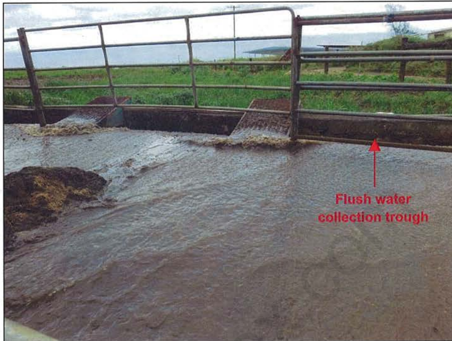
Photograph 13. Flush water from the 380-head calf barn is captured in a collection trough located at the end of the barn and conveyed to the manure composting building collection pit, shown in Photographs 15 and 16. Photo by A. D'Angelo; 12/14/16.
