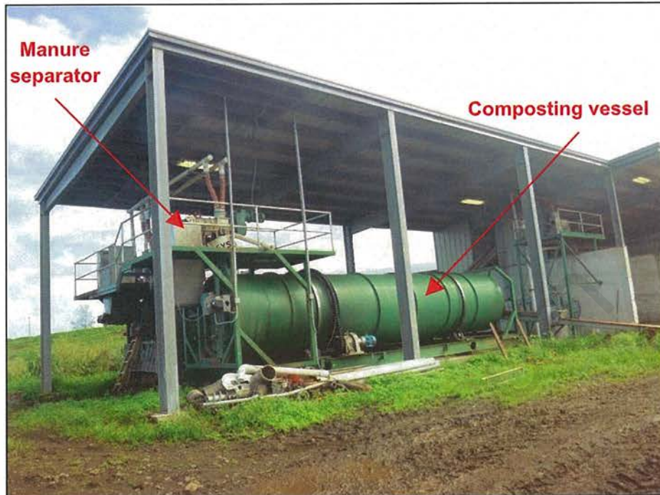
Photograph 17. View of the Facility's manure composting building which included two manure separator units, and two composting digester vessels. Photo by A. D'Angelo; 12/14/16.
